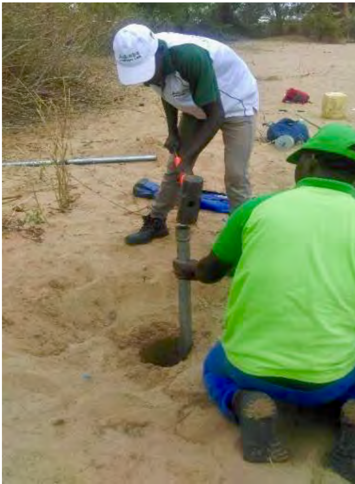
Figure 2: Bailing method of drilling wells.
