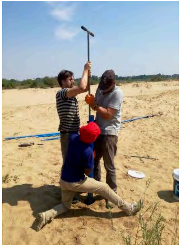
Figure 3: Driven well-point method of drilling wells.
