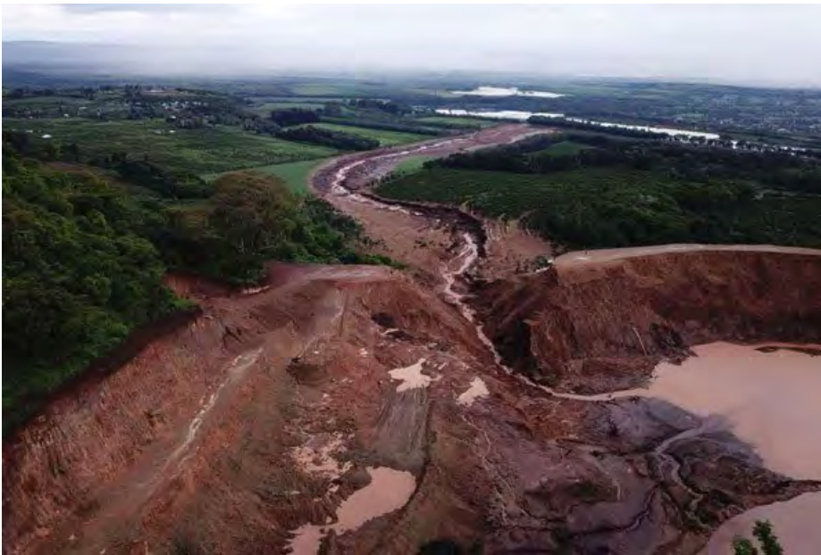
The Patel Milmet Dam was a privately owned embankment dam located near the township of Solai, Nakuru County, in Kenya's Rift Valley. The dam burst amid heavy rains on 9 May 2018, killing at least 48 people.
